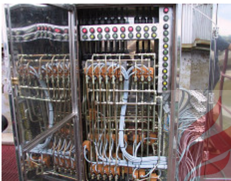
Hydraulic and electric control panel of vertical and horizontal pig-launcher stations
