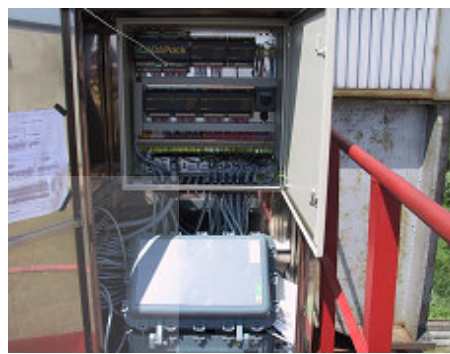
Hydraulic and electric control panel of vertical and horizontal pig-launcher stations
