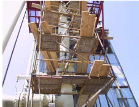
Testing of vertical pig chamber by manufacturer
